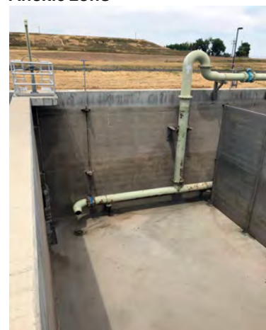
Figure 4-14: Internal Mixed Liquor Recycle Header
