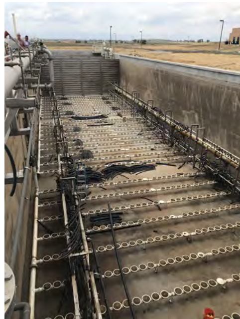
Figure 4-16: Removal of Heat Exchange Coils
