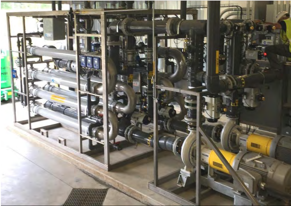
Figure 5-16: Typical Pressurized UF Configuration
